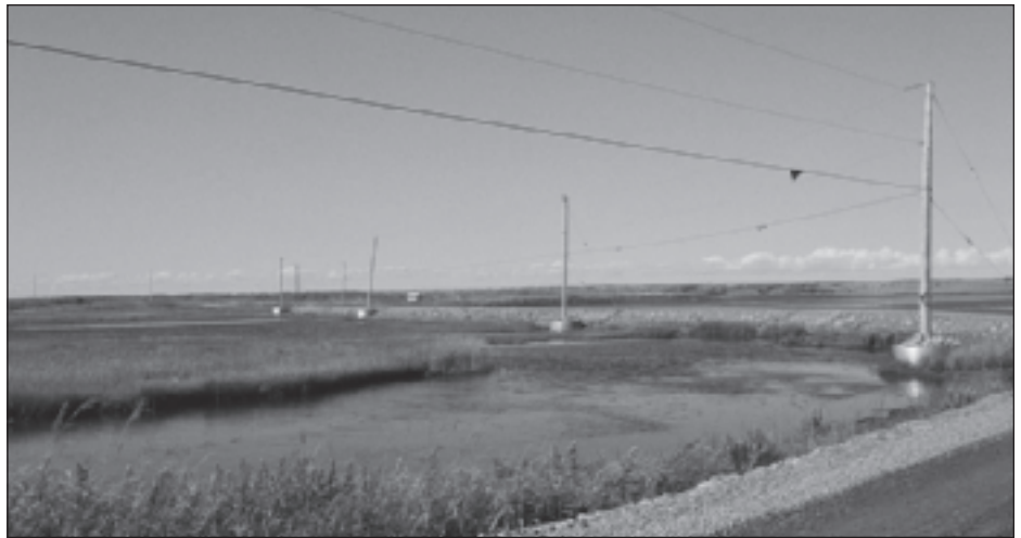
The causeway to Delorey Island is vulnerable to flooding.
